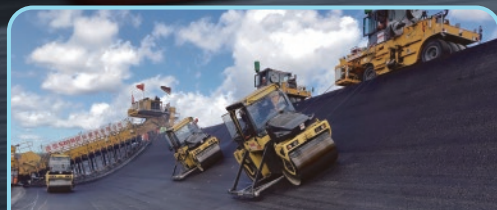
T1: Asphalt concrete high-speed track with the largest inclination in the world
